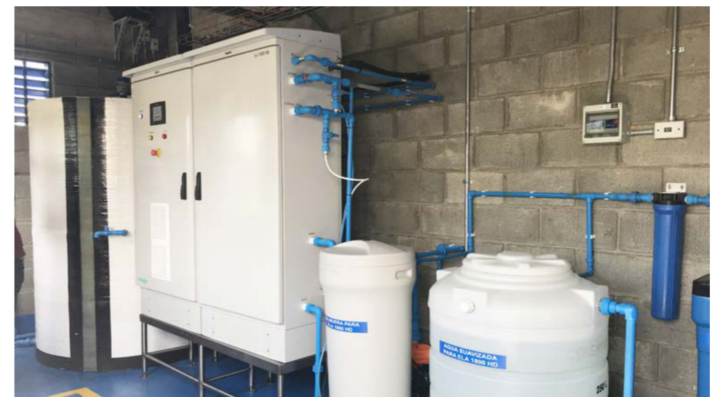
ELA 1800HD set for 5000ppm for public water treatment
